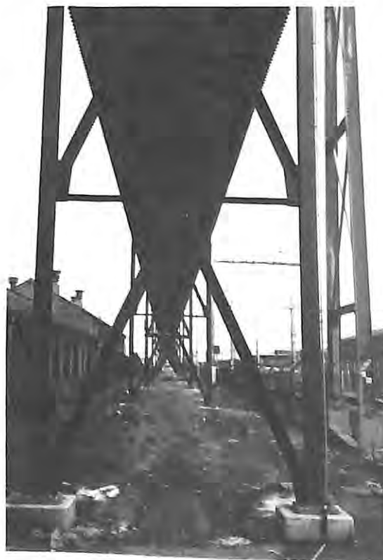
This red and white coal conveyor travelator brings imported coal under the River Avon at Avonmouth to a ginormous hopper under which coal trains move at creeping pace to be loaded. The Avonmouth area is the most impressive industrial area in the southwest of England. Photo by the editor 1994
